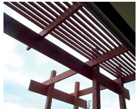
Example of pergola structure within building envelope.
