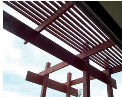
Example of pergola structure within building envelope.
